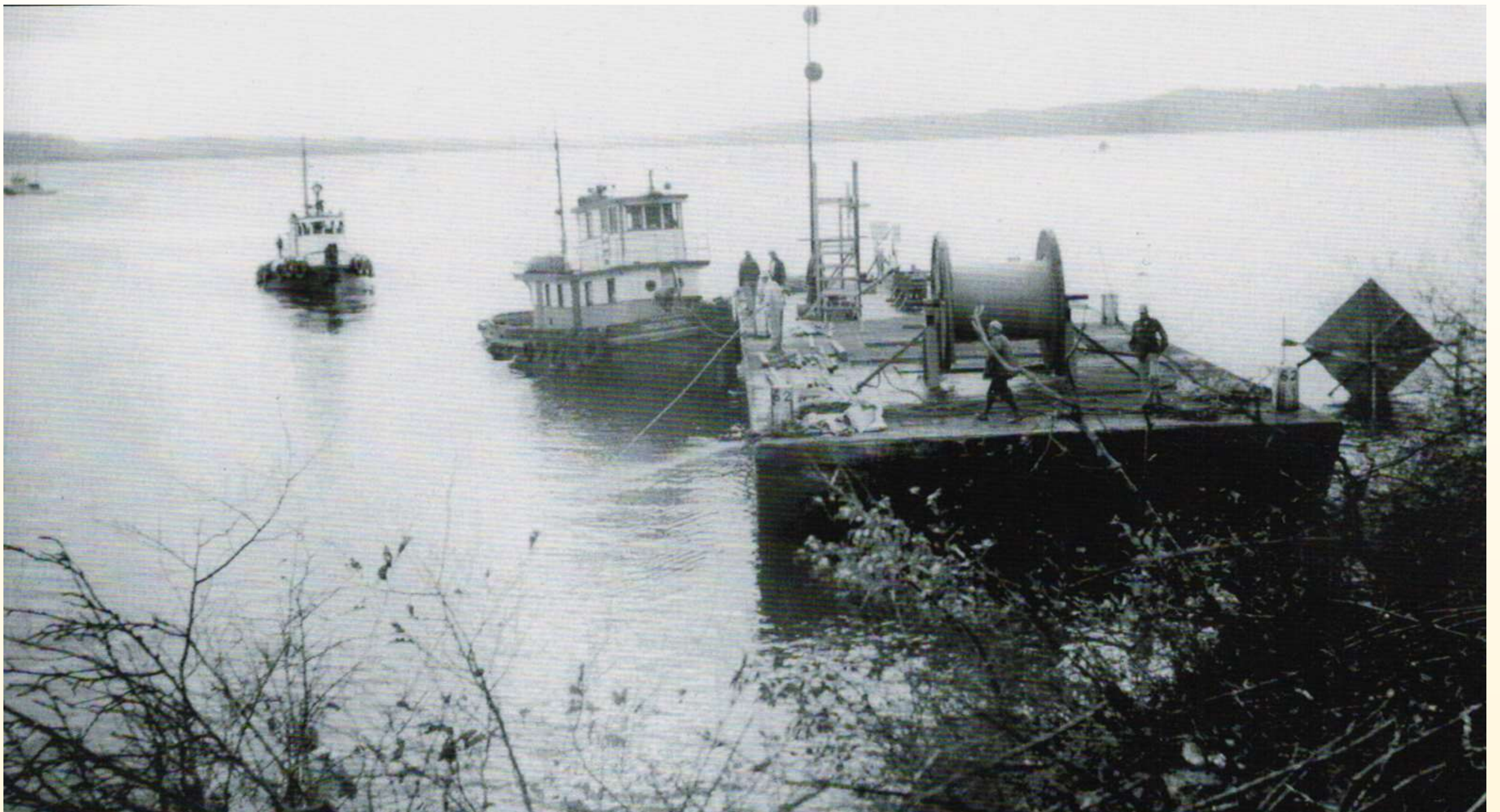
Laying the 2 mile cable from Nisqually Reach to the south end of Anderson Island, October 1961.
